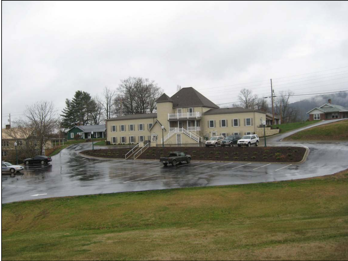
Figure 3. Photograph of Mars Hill Town Hall, site of the LID demonstration project.
