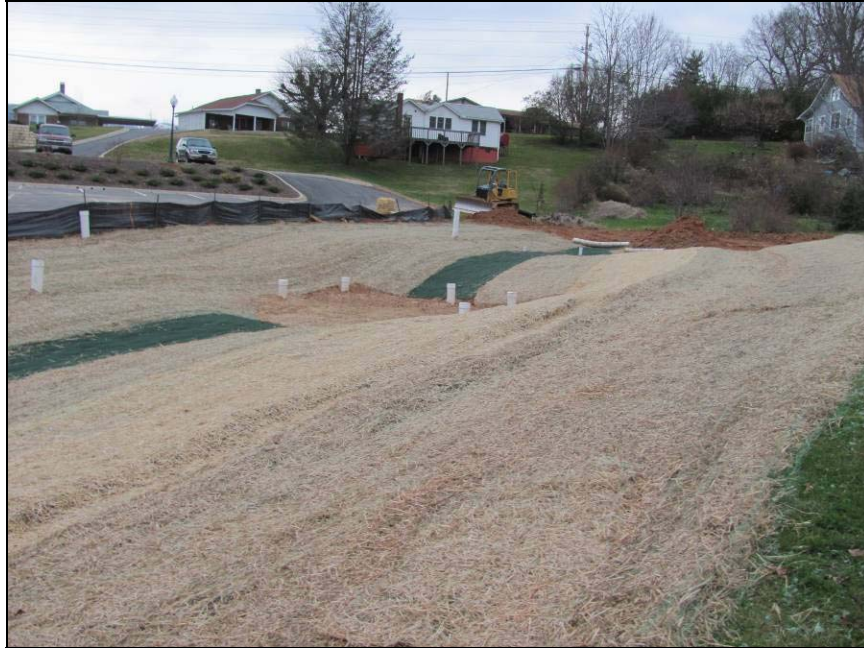
Figure 8. Mars Hill LID demonstration project site under construction.
