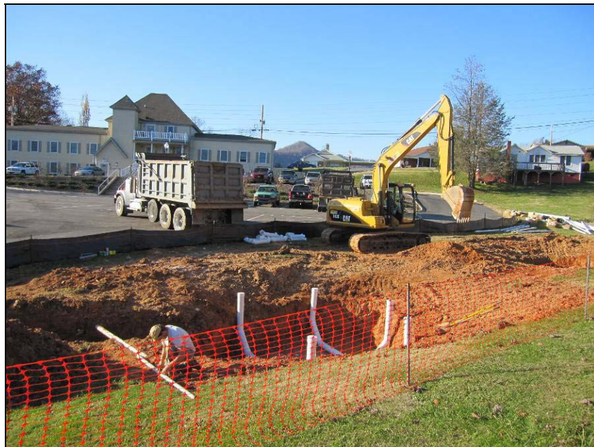
Figure 7. Mars Hill LID demonstration project site under construction.
